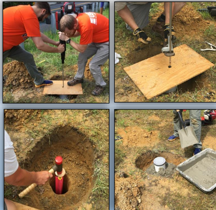
3-D Deep Rod Installation at Jamestown, VA
