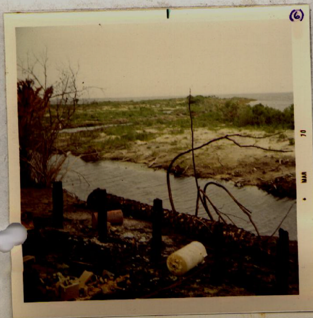
(6) Point of land that has been ditched and drained, now being above mean water level for the most part.
