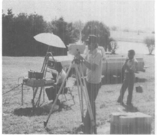
Figure 4.—Leveling team in operation.
