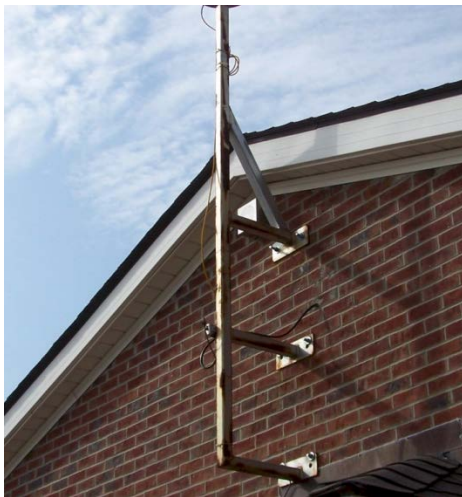
Figure 2 - Outrigger Mount
