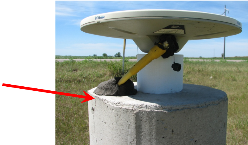
Figure 5 – view of pillar monument (note the crack that has developed near conduit location)
