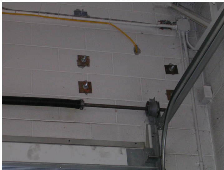
Figure 4 – Through-bolts with backing plates
