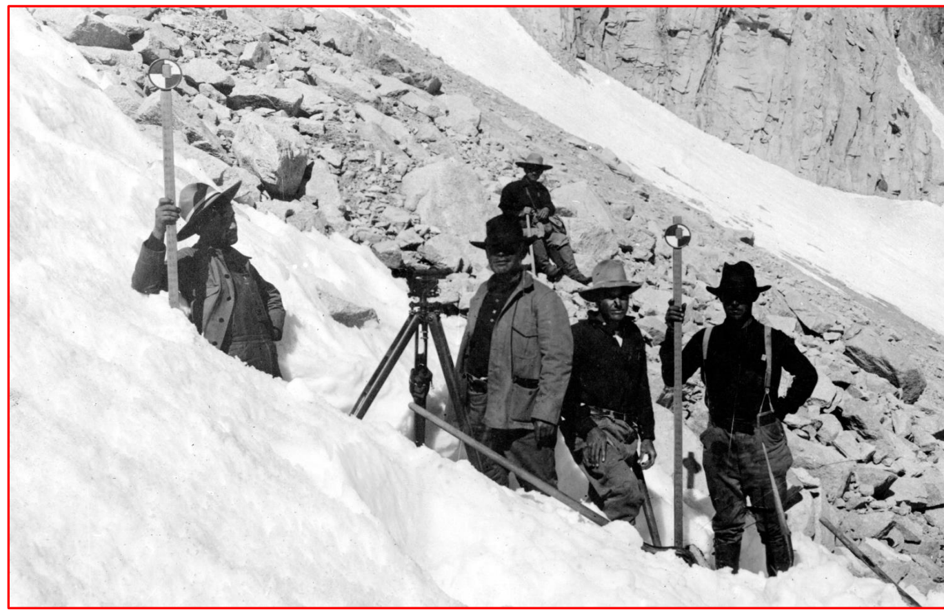
Figure 1. 1905 U.S. Geological Survey leveling party surveying in arduous, high-elevation conditions on Mt. Whitney, Sierra Nevada, CA.
