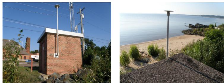
Figure 3. WLS and collocated CORS (MIMQ) in Marquette, Wisconsin. Distance was measured from CORS ARP to the Electronic Tape Gauge (ETG) on the bench in the structure. Drops are made from the ETG table to a well freely connected to the water surface. When the sensor hits the water and completes an electric circuit, the distance is recorded. This provides a means to transfer the water level surface into geometric coordinates.
