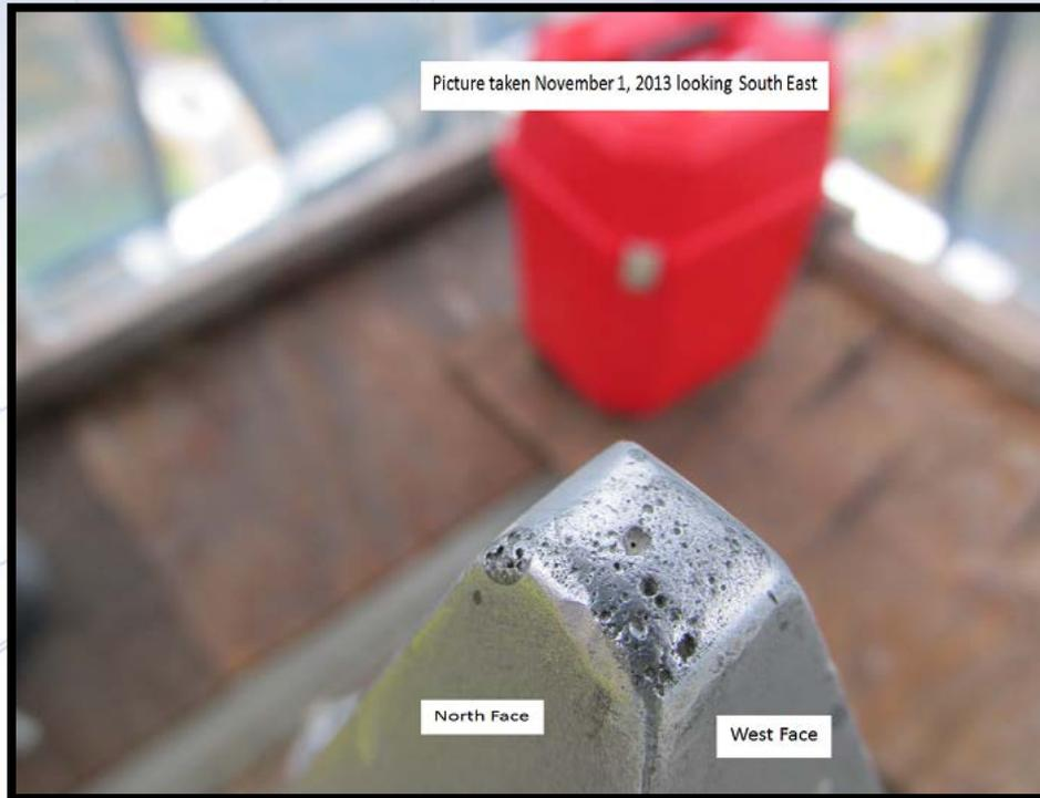
The only observed source of any structural loss of architectural height is from rounding of the tip of the monument, amounting to  $\frac{3}{8}$  of an inch.
