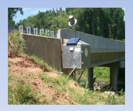
GPS and traditional leveling will be use to connect stream gages to NAVD88
