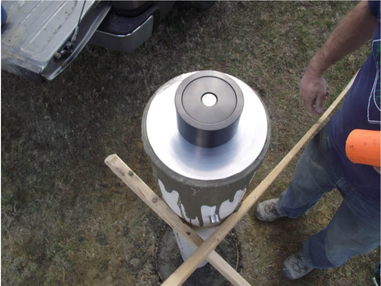
Figure 12. Fine leveling of the adapter. Using a precision bubble level, fine level the top of the forced centering adapter by gently tapping on the top sides. Leave the braces in place for at least two days before removing them.
