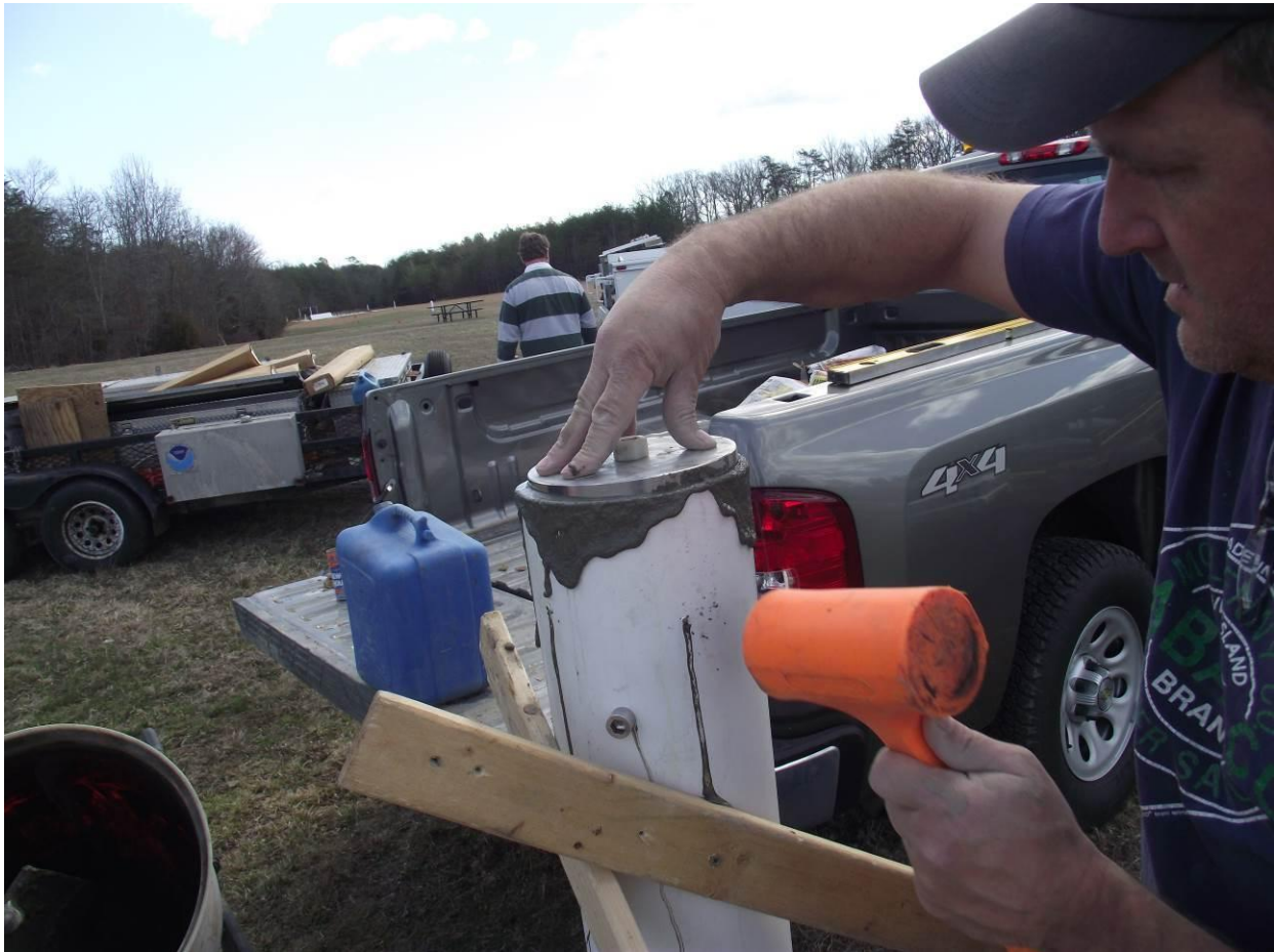
Figure 11. Install the forced centering adapter. Insert the forced centering adapter into the top of the PVC pipe tapping sides of the pipe with a hammer until the top of the adapter is fully seated. Ensure there is no air gap between the bottom of the adapter and the concrete inside the pipe.
