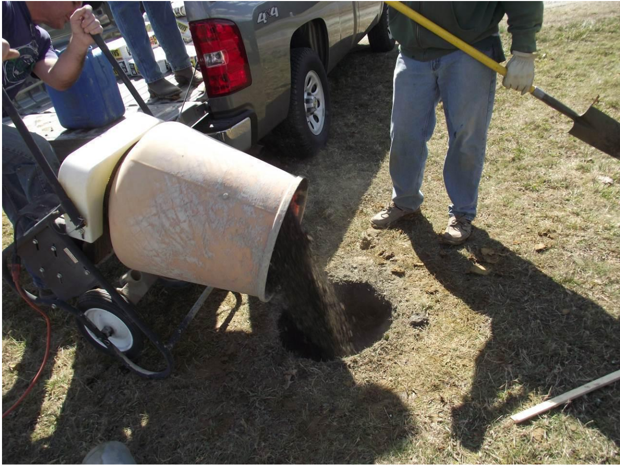
Figure 7. Filling the hole with concrete. After having drilled the 18-inch diameter hole to a depth of 10 feet and tamping any loose soil in the bottom, fill to within 1½ feet of the top of the hole with 3,500 PSI synthetic fiber reinforced concrete. Use a vibrator to consolidate the concrete. Insert the 1½ foot-long section of 18 inch diameter cardboard form into the hole.
