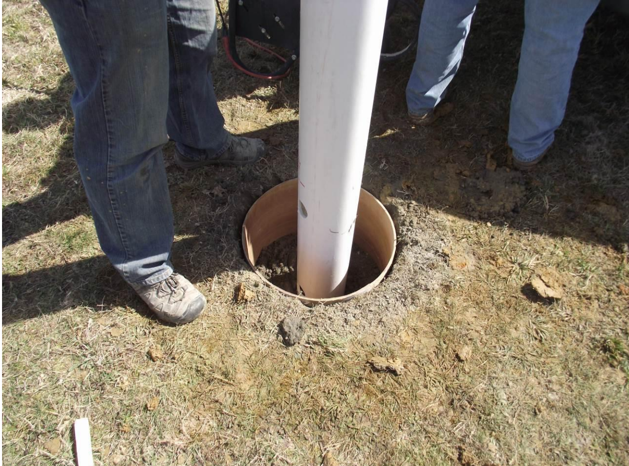
Figure 8. Position the PVC pipe at the desired location in the drill hole. Mark the PVC pipe at 2 ½ feet from the bottom. Insert the PVC pipe into the hole until the mark on the PVC pipe is at the same level as the top of the form.
