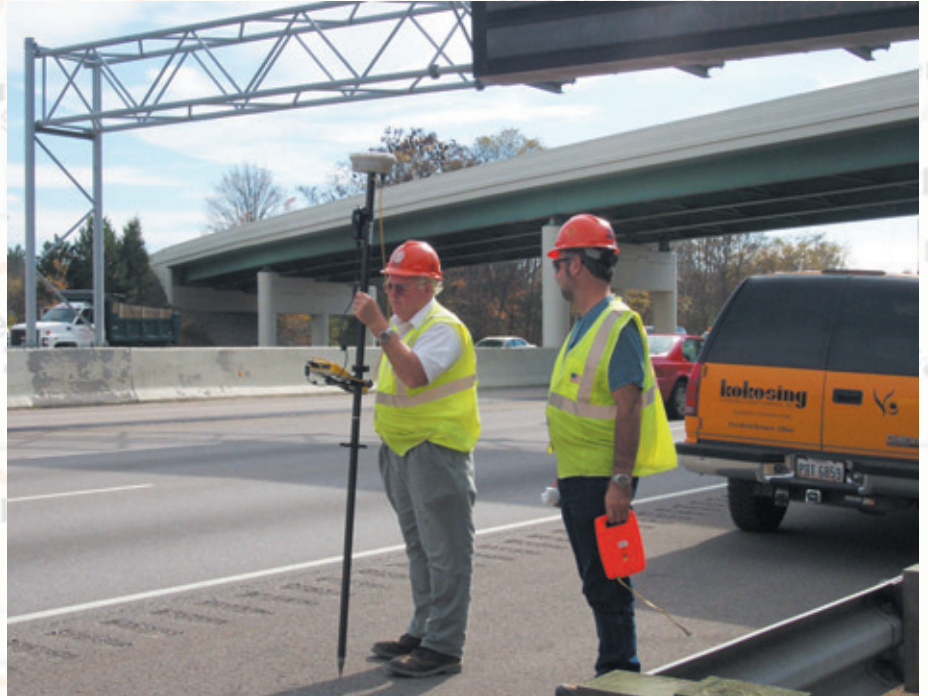
Kokosing Construction Co surveyors Rex Bogner and Dan McIntire do sign layout using a Trimble 5800 RTK GPS system with the ODOT VRS Network on an I-71 ODOT project.
