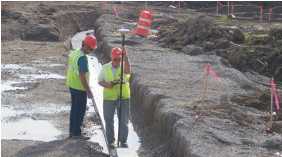
Kokosing Construction Co surveyors Rex Bogner and Dan McIntire as-built MSE wall footers using Trimble 5800.
