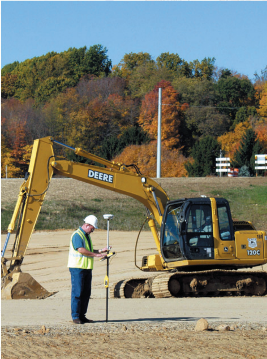
ODOT CORS Construction Manager/Surveyor David Beiter surveys newly constructed sub-grade for US33 Lancaster Bypass project in Lancaster, Ohio. Image courtesy: Chuck Bernthold
