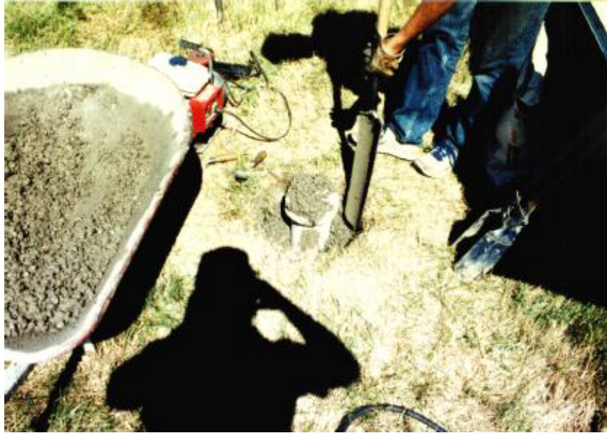
Backfilling Remainder of Hole with Concrete
