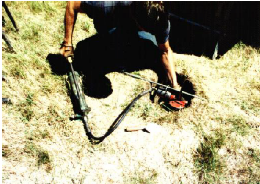
Cutting the SS Rod 3" Below Ground Level with Hydraulic Cutter
