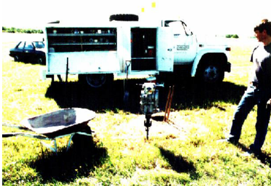
Mark Setting Truck and Equipment
