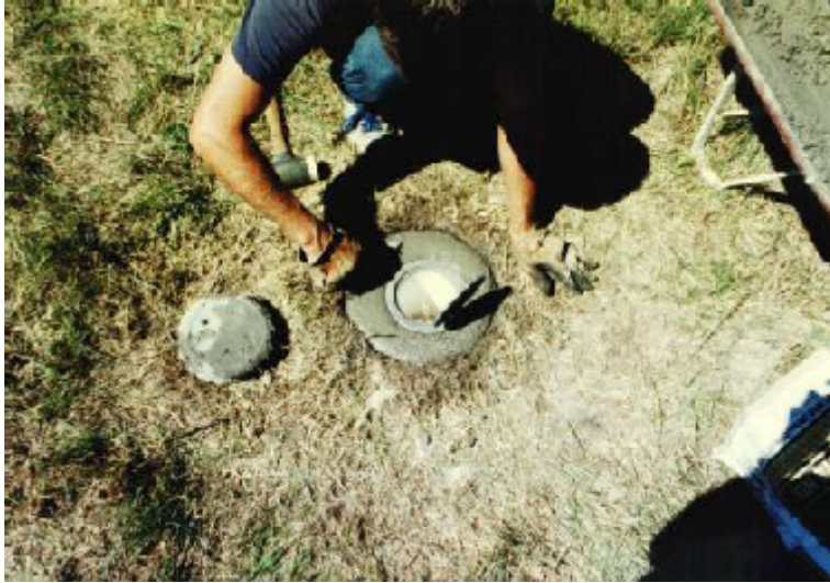
Trowling Smooth Top of Concrete Note, No Concrete on top of Logo Cap
