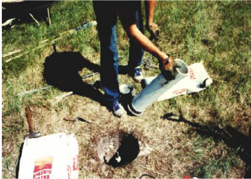
Gluing Logo Cap to 5" or 6" PVC Pipe
