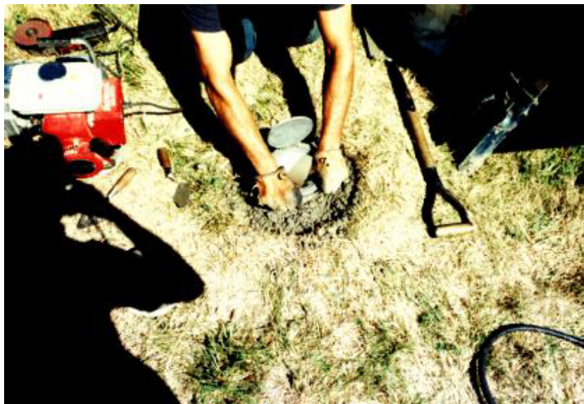
“Shaking” PVC Pipe to Help Settle Concrete
