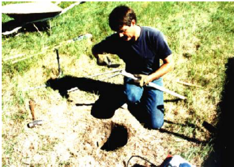
Preparing 1" PVC Greased Filled ("Finned") Sleeve
