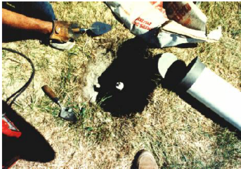
Preparing Hole For 5" or 6" PVC Pipe
