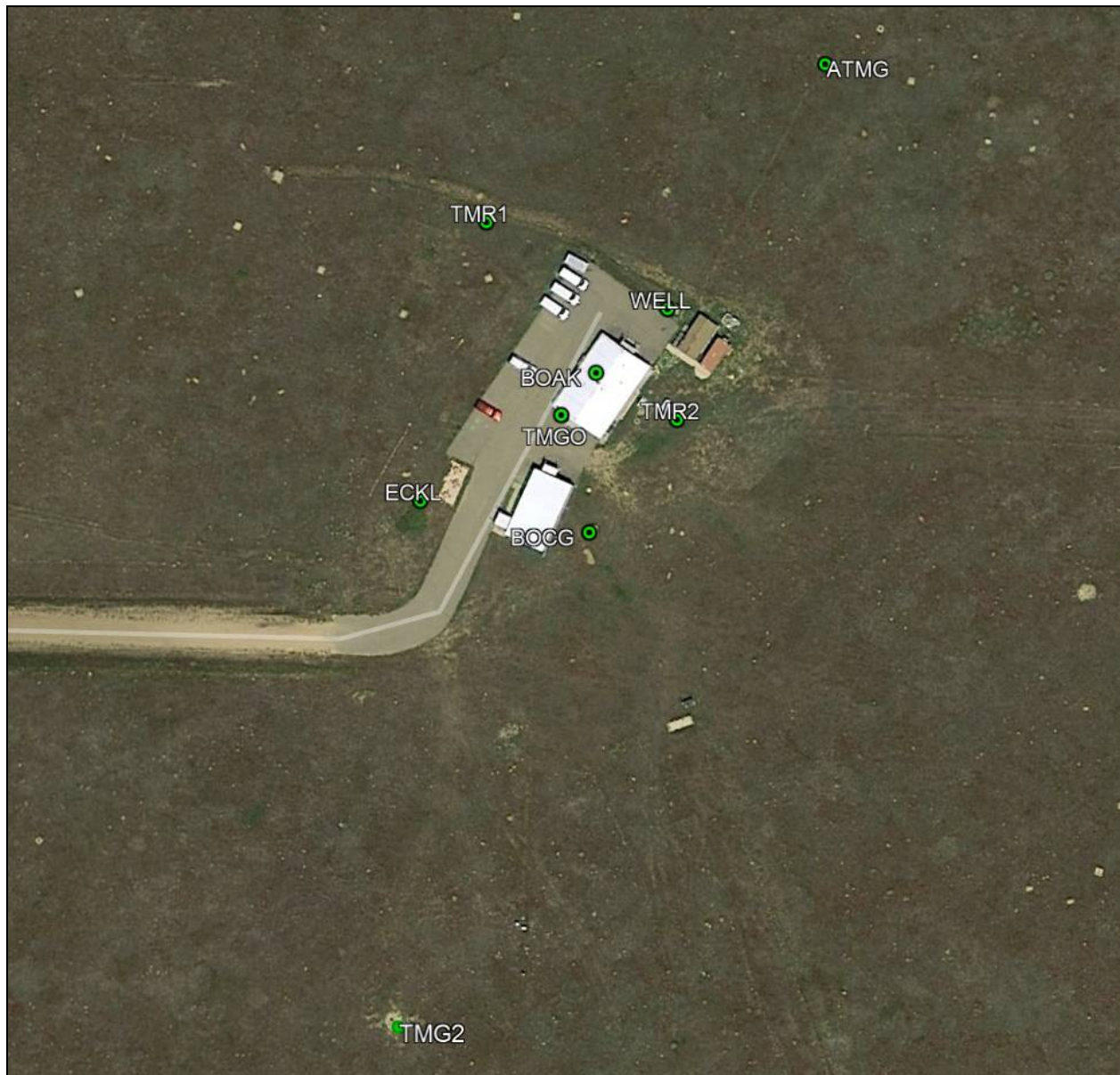
Control stations at Table Mountain Gravity Observatory
